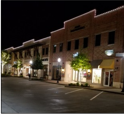
Downtown Lighting - Project 2.2
