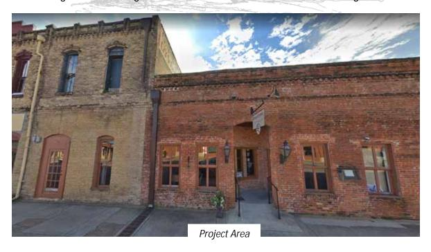
The existing windows are two over two double hung wood windows. One window on the second story was at some point replace by a door. These will all be replaced with Pella Architectural Series, two over two, wood double hung sashes with Enduraclad exterior with an Auburn brown finish (Attachment 1). The brick sill will be rebuilt on the second story window that is currently a door.
