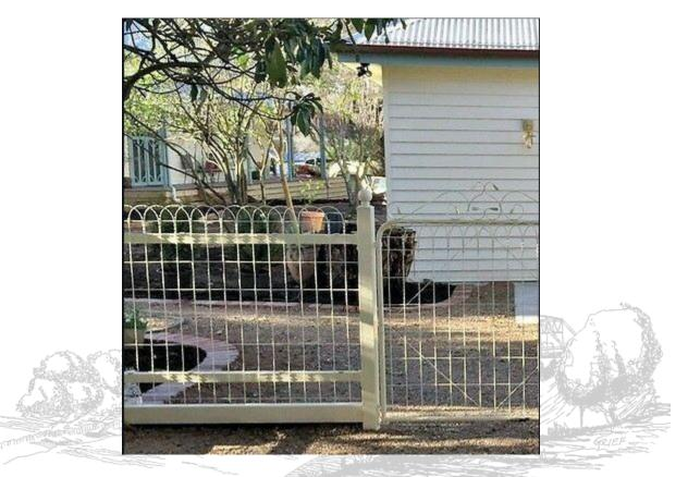
The applicant has already begun installing the fence with the wooden support, shown below (Attachment 5). There will be a 2-inch by 4-inch cross support added along the bottom.
