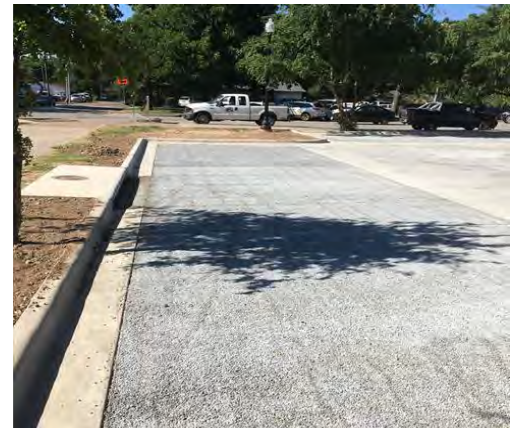
Parking lot at Alley D
