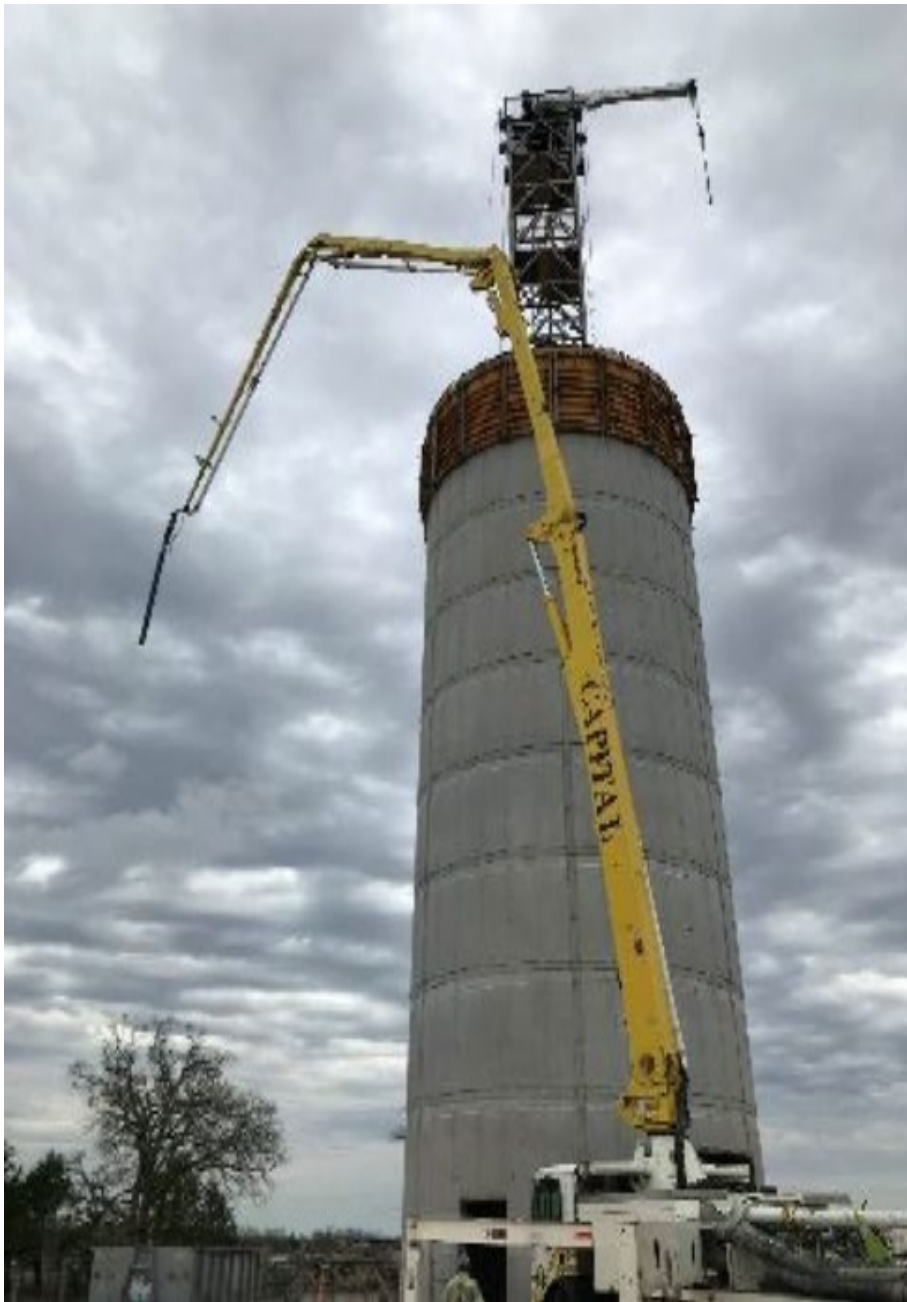
Placement of Lift #10
