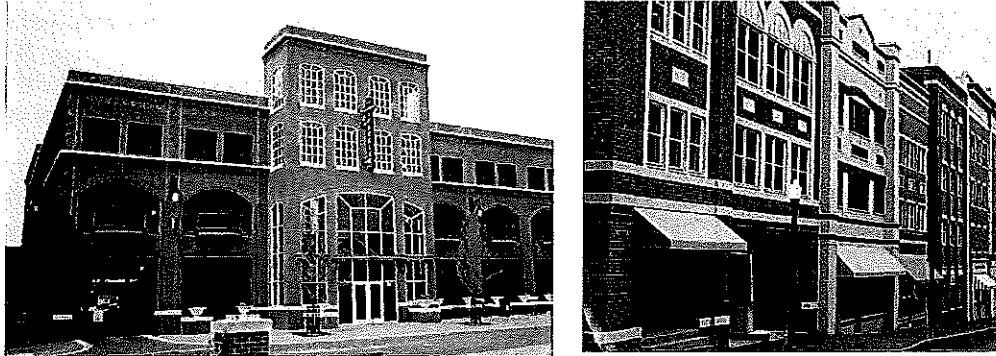
Figures 7-13 Images showing required façade treatment of parking garages along Primary Frontages
