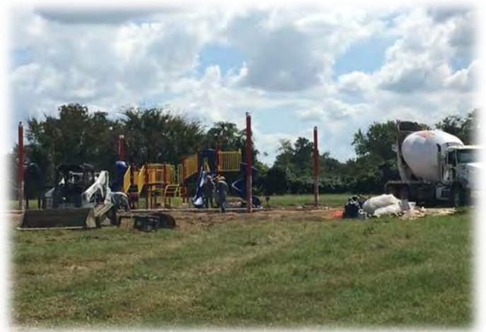
Picture: Delgado Park under construction
