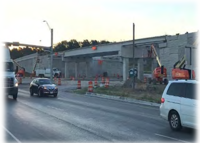
Picture: SH 71/95 Interchange under construction
