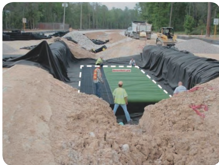
Underground storage tank, Birnamwood Drive
