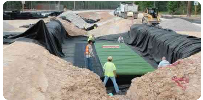
Bioswale and Underground Storage Construction, Birnamwood Drive
