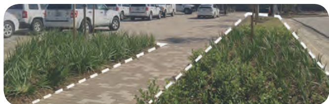
Bioswale, Houston Permitting Center
