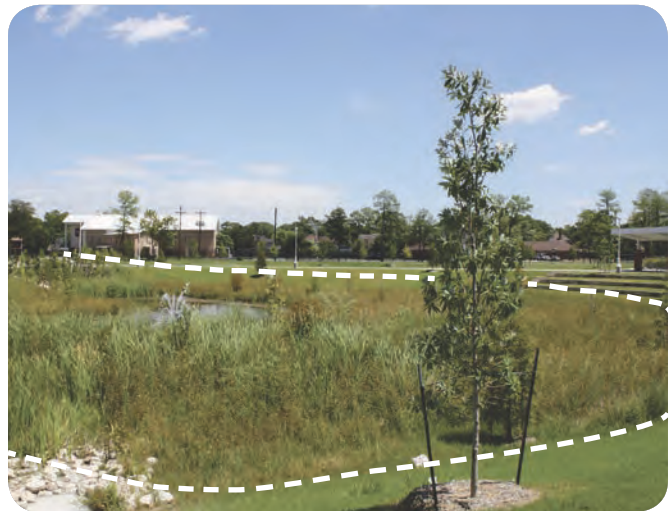
Vegetated Filter Strip, Lone Star College Victory Center
