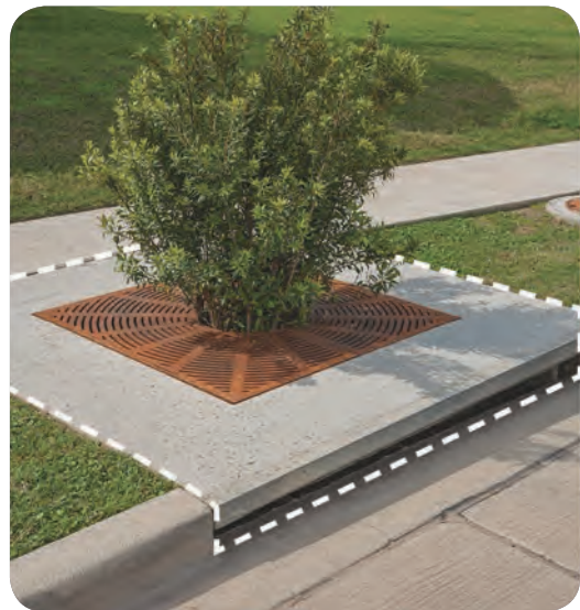
Stormwater Planter Box, Darling Street
