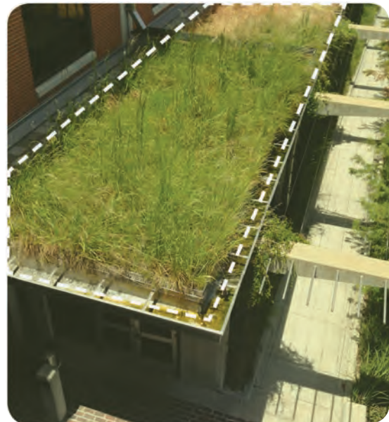
Green Roof, Houston Permitting Center
