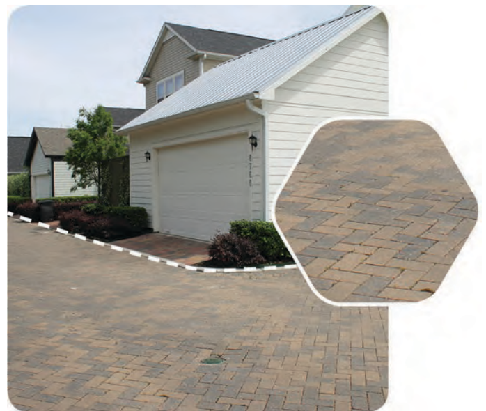
Permeable Pavement, Kempwood Manor
