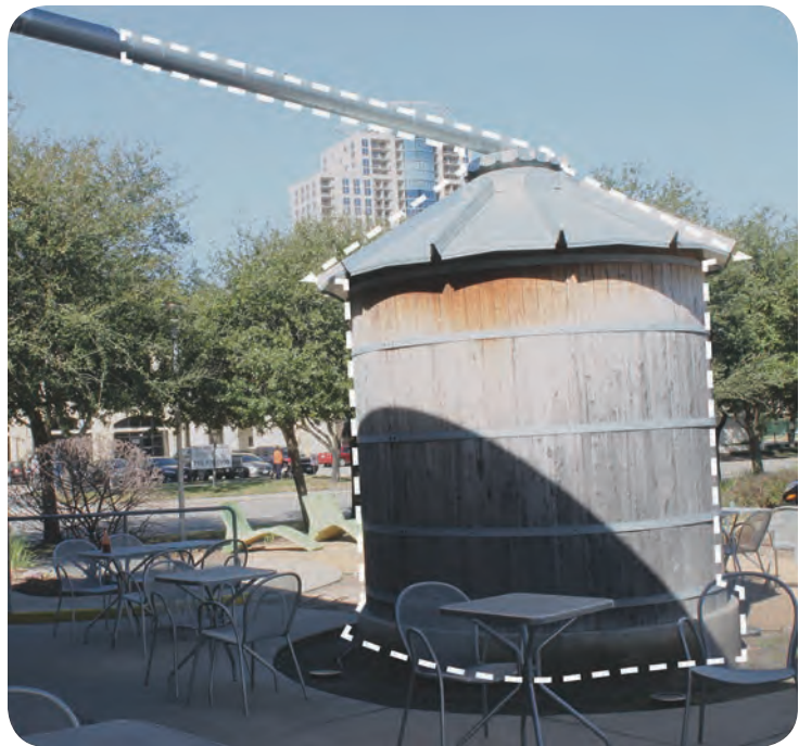
Cistern, Grocery Store in Houston
